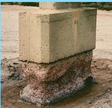
Pipeline support chair cast in 1960 with ordinary concrete after 2 years
